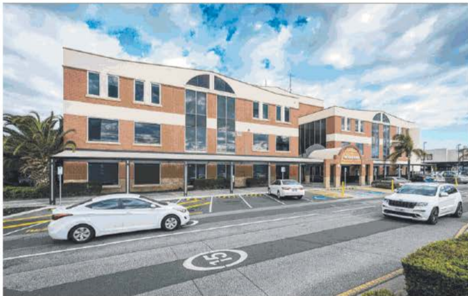
A 100kW solar system is set to be switched on at Port Adelaide's Custom House next month.
